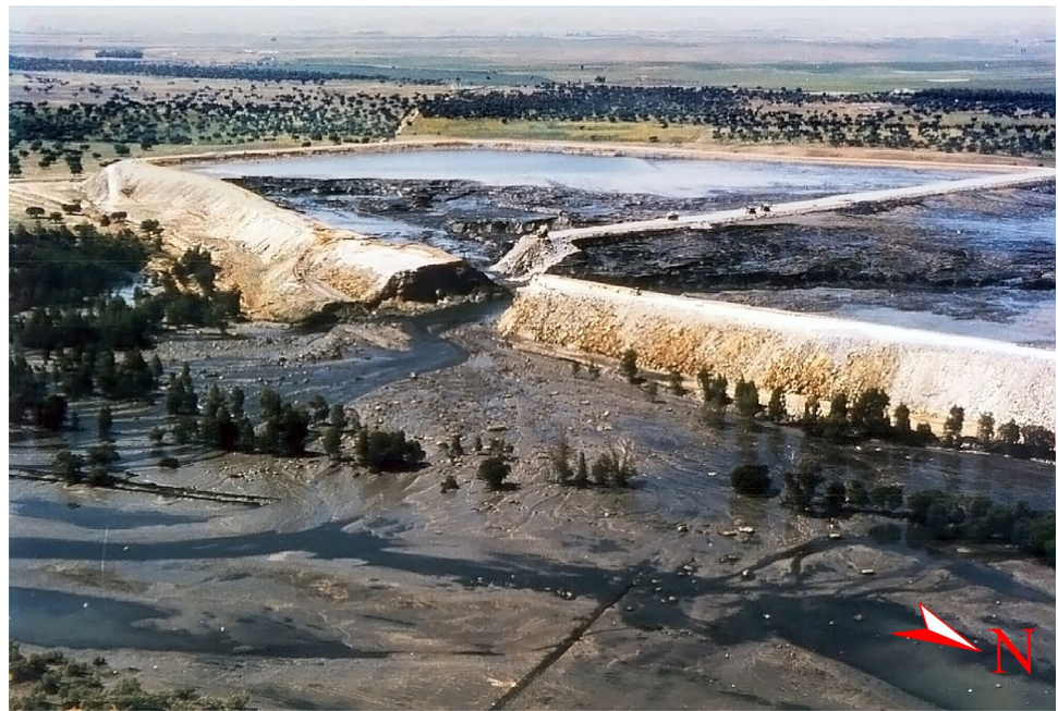
Fig. 3 April 25, 1998; early morning. On the left, the displaced stretch of the dam and the opening allowed a fraction of the stored tailings and water to spill out, north and south of the transversal dyke. The original breach was estimated at about 14 m wide. Subsequent erosion increased the gap to about 25 m
